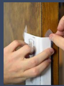
Using a sharp object (like a nail, thumb-tack, or drill bit) mark the two 10mm (1/8") holes and the 25mm (1") hole to be drilled.
