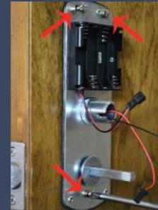
Tighten the fixing bolts. Test the spindle again. Do not overtighten the bolts as this may cause the door to distort and affect the lock function.
