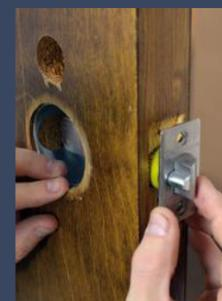
Insert the latch with the bevel towards the door frame and secure with screws.
