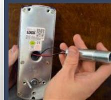
Screw the cable tube into the front plate (slotted side out), passing the cable through the tube.
