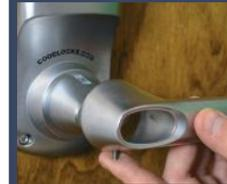
Fit the key cylinder plate over the key cylinder. Then install the front handle.
